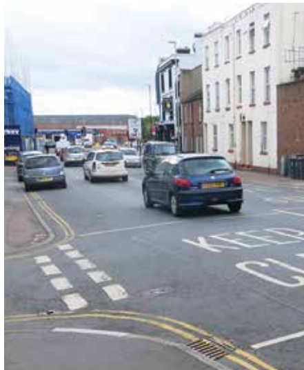
Existing Secondary Street context
